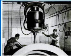
The G-E million-volt X ray cuts from hours to minutes the time required to examine metal parts—from airplane crankshafts to turbine shells.
