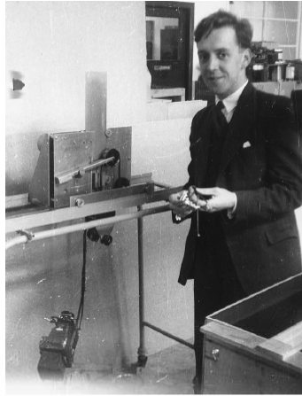
Fig. 3. Tom Brown with the first contact scanner in the development laboratory at Kelvin Hughes Ltd., Glasgow, 1957. This machine commonly is referred to as the "bed table machine," as a hospital bed table was used to support the scanning mechanism. (From BMUS Collection.)
