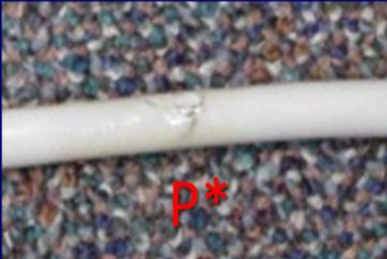
Partial Cable Tear
